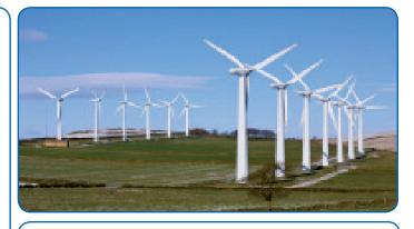
58% due to more favourable wind regimes than other areas in the Europe<sup>(7)</sup>. \*Capacity factor = Actual amount of power produced over time / Power that would have been produced if turbine operated at maximum output 100% of the time.
